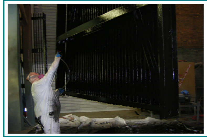
Application of black silicone Top Coat
