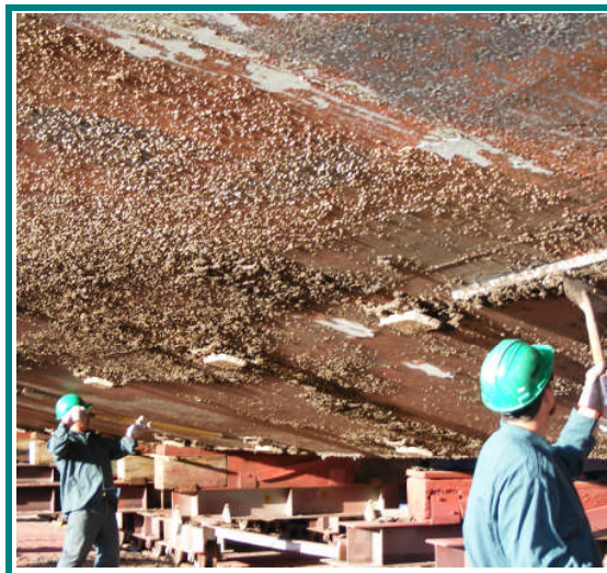
Cleaning fouling growth from bottom
