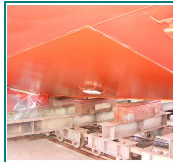
Completed test patch close-up
