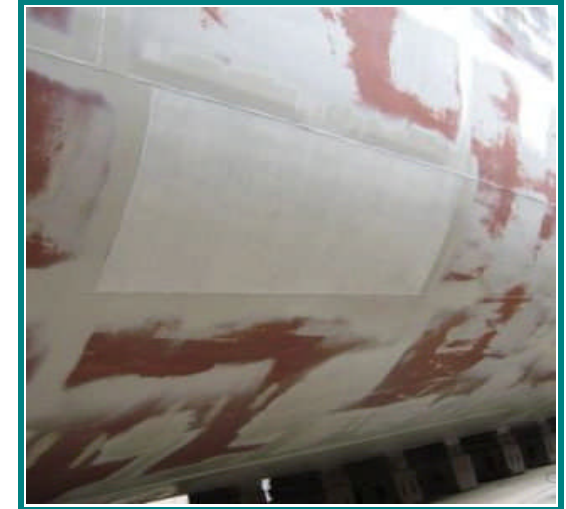
Completed test patch close-up
