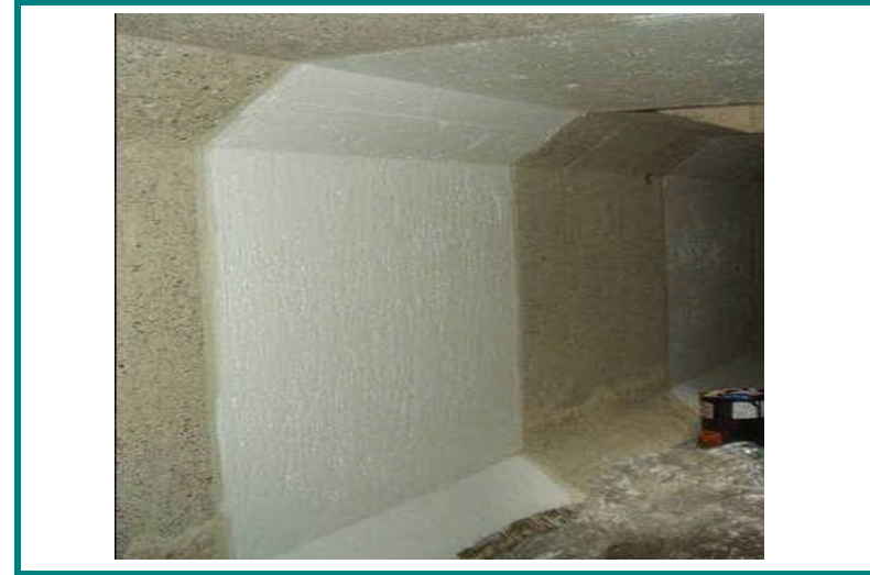
Completed test patch in Unit #6 intake tunnel
