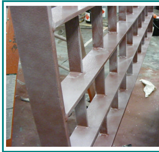
Completed silicone Tie Coat
