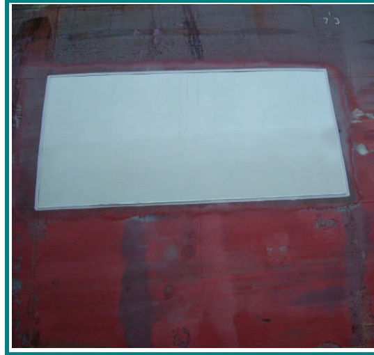
Completed test patch full view
