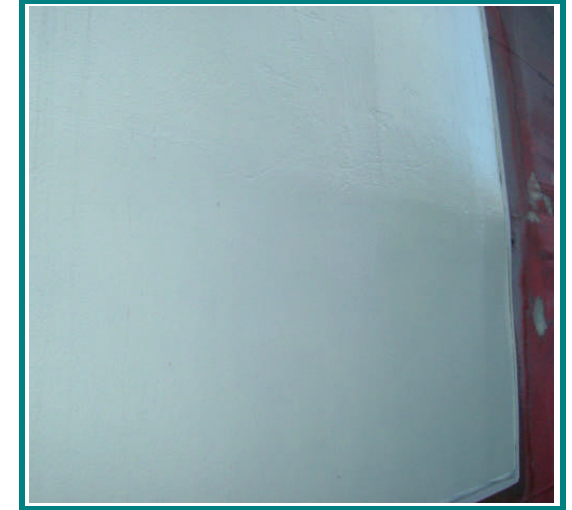
Completed test patch close-up
